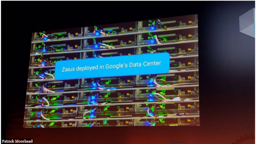
Patrick Moorhead Google announced it has deployed POWER-based systems into its data center
